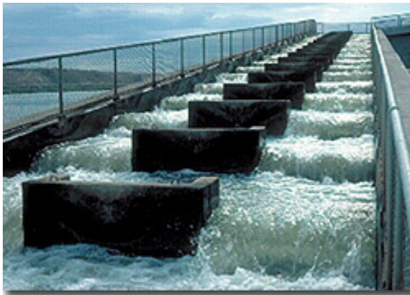
Fish ladder at Ice Harbor Lock and Dam North on the Lower Snake River, WA. (Photo: US Army Corps of Engineers)
